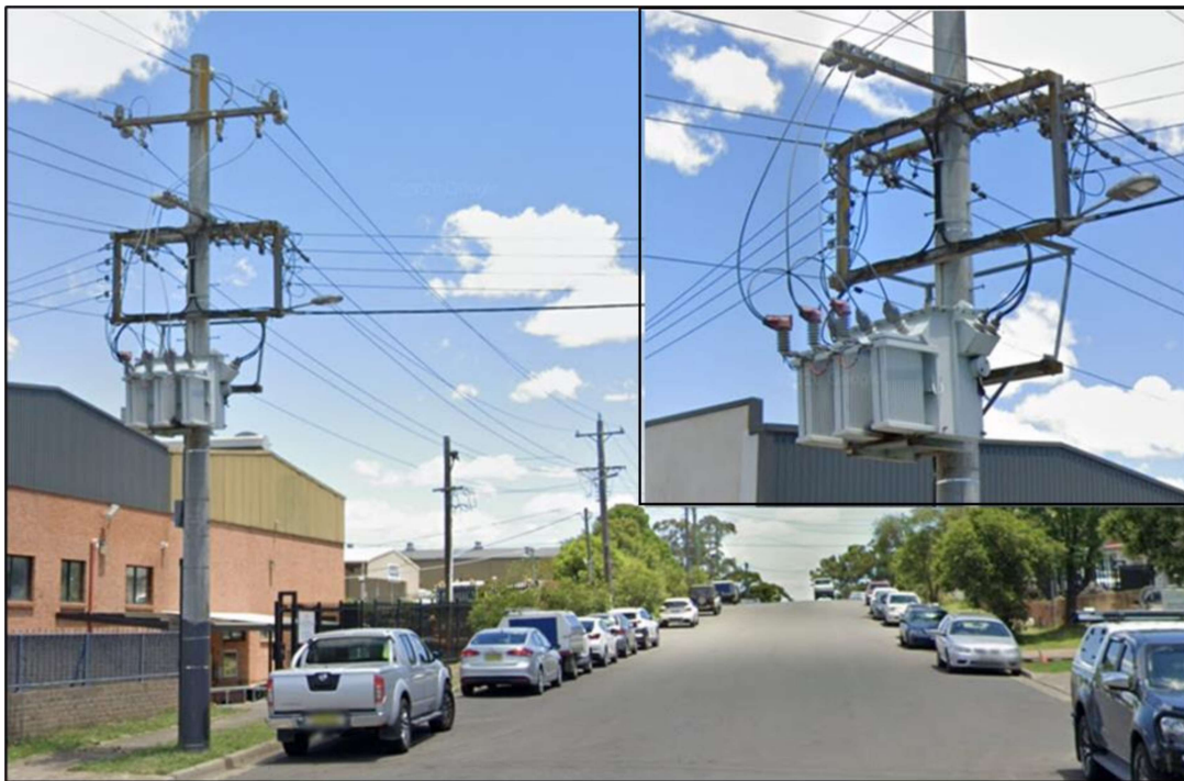
Pole mounted substation in Wellington Street Riverstone. Source: Google Maps Street View.
