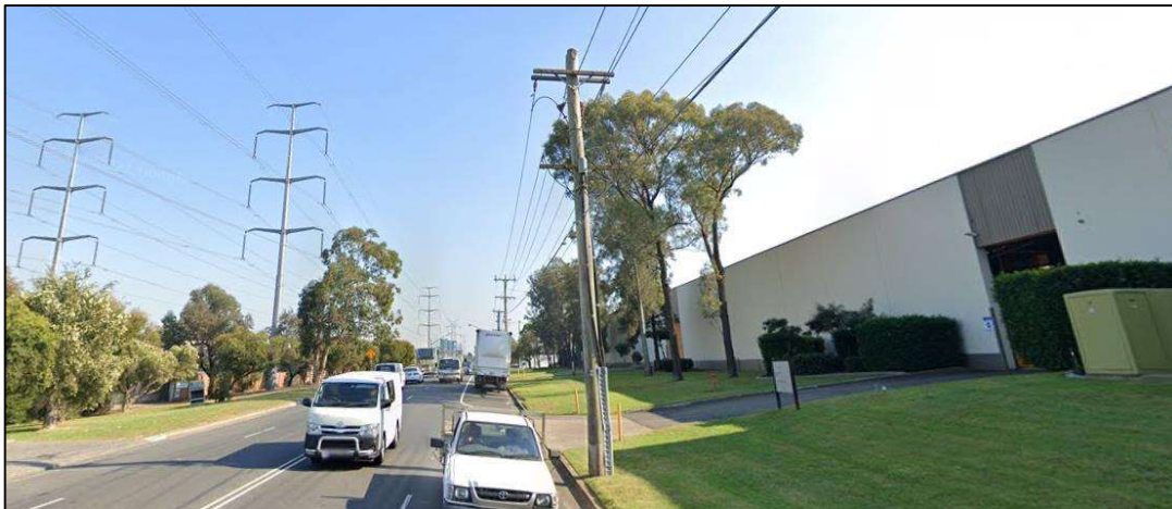
Transmission, high voltage and low voltage overhead power lines in Long Street Smithfield. There are also high voltage underground cables coming from the pole going to the padmount substation. Source: Google Maps Street View.
