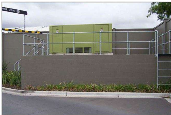
Figure 51 - Example substation raised above 1:100 flood level
